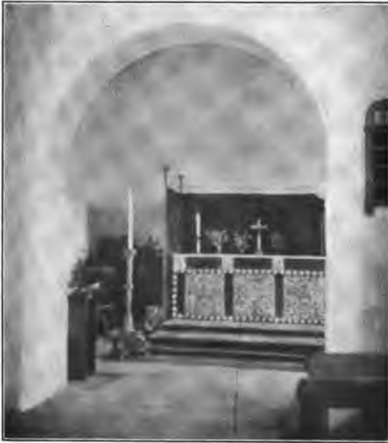
Chancel Arch of the Village Church, Caldey Island
