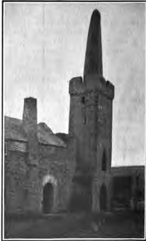
The Priory Tower and Gateway from the Exterior
