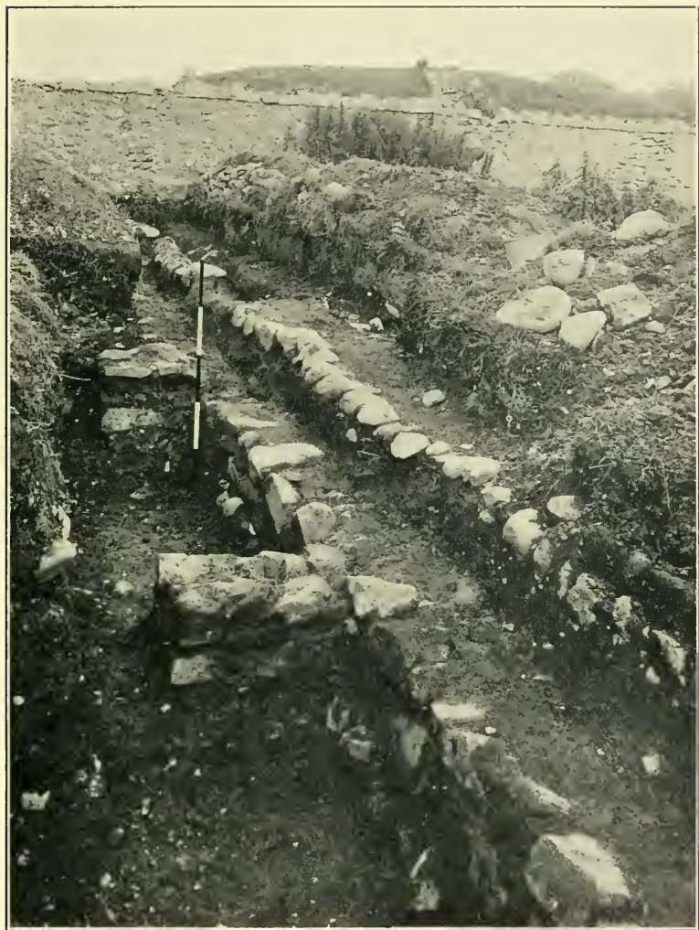
Fig. 7. Buttressed wall of building XXI, with footings of fourth-century wall at higher level.
